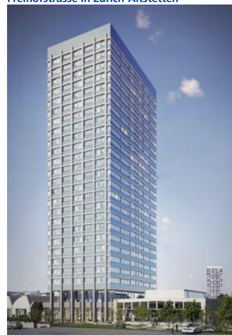
Figure 3: Residential tower "ALTO", Freihofstrasse in Zurich-Altstetten
