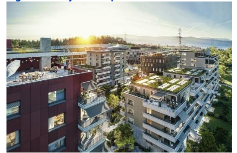
Figure 2: Project completion in Cham
