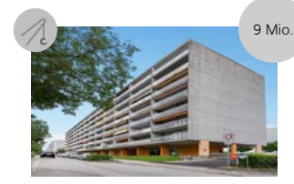
Boudines, Meyrin Energy renovation
