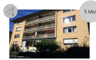
Contigny, Lausanne Renovation & extension
