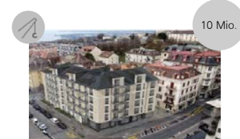
Jomini, Lausanne Renovation & extension
