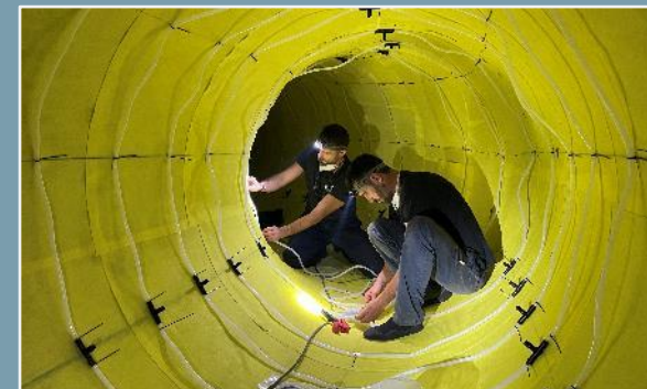
Water pipes retrofit/repair with composite materials
