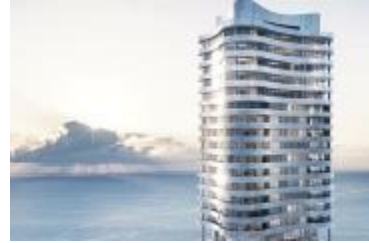
Hedges Ave Residence, Gold Coast (Australia)
