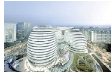
Galaxy Soho Office Building, Beijing (China)
