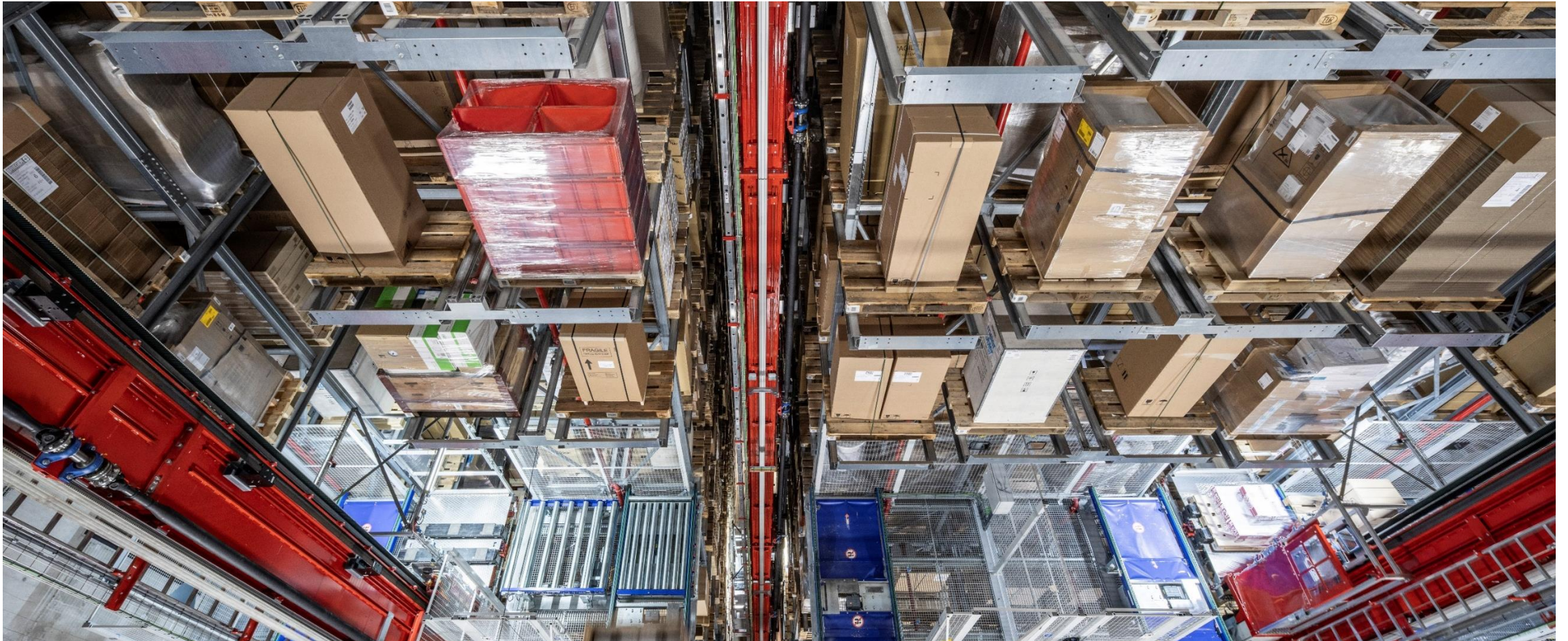
Five storage and retrieval machines access the HBW at speeds of up to 22 km/h, 30 metres high
