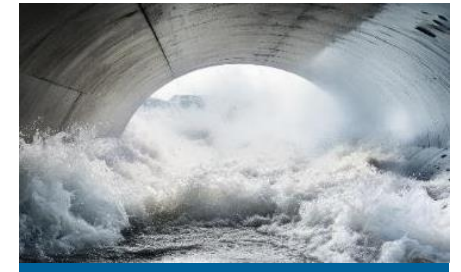
Waste & Storm water management
