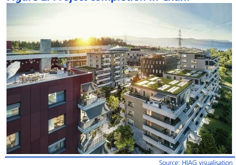
Figure 2: Project completion in Cham
